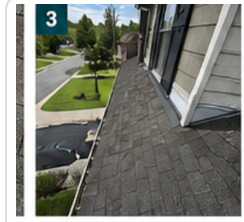
SHINGLE DISPLACEMENT
