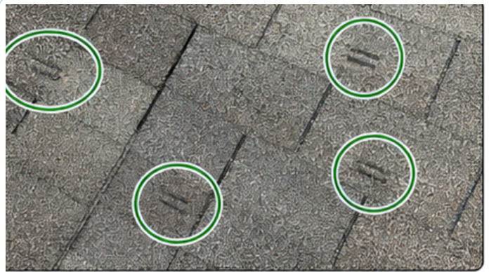
Repeated wind-stress indicators on field shingles
