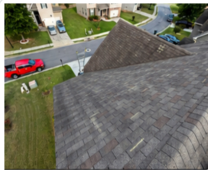
Directional uplift pattern DIRECTIONAL UPLIFT PATTERN
