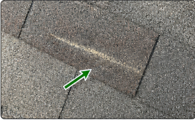
Directional creasing along shingle tab
